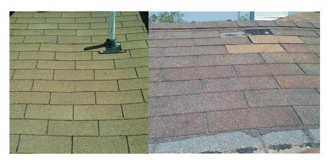
Roof deck has areas of failure as evidenced by undulations in roof.
