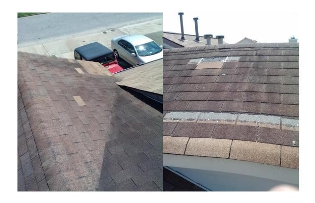
Roof shingles are beyond their operable age. As evidenced by extensive patching, missing shingles, breaking, and exposed nail heads. Replacement is recommended
