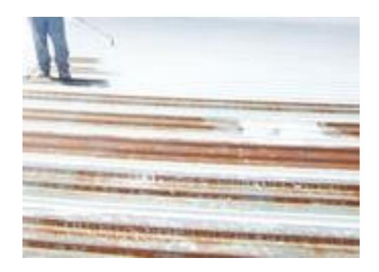
Application of two coats of Astec primer B-16-71 rust inhibiting primer.
