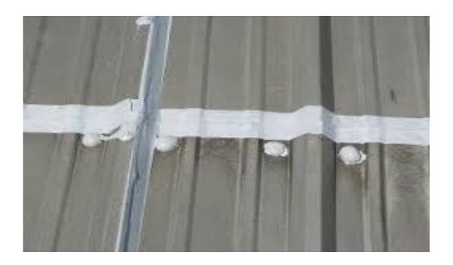
Vertical and horozontal seams to be waterproofed utilizing 4" tape and WPM#9 caulk. Roof penetrations to be flashed using Astec WPM#10 Fibered Caulk
