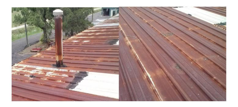
Pressure clean roof panels, wire brushing areas with advanced stages of corrosion, and patching or replacing panels where rust has eaten completely through the roof panel.
