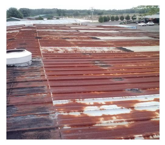
Roof has reached the end of operable age. Recommend roof restoration.
