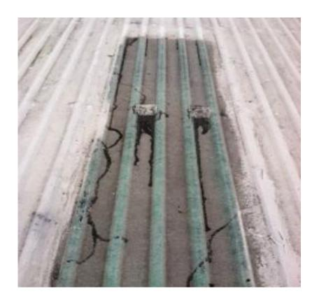
Restoration of existing skylights using ASTEC Skylight Sealer. The ASTEC skylight sealer is a clear acrylic formulated to renew the appearance of aging skylights while protecting the light from moisture and ultraviolet degradation.
