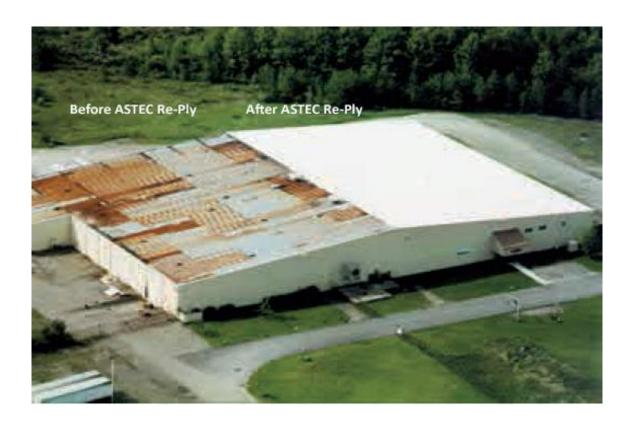
Application of 12 mils of ASTEC #2000 Finish coat to entire roof area; and issuance of a 10 year Labor and material warrant
